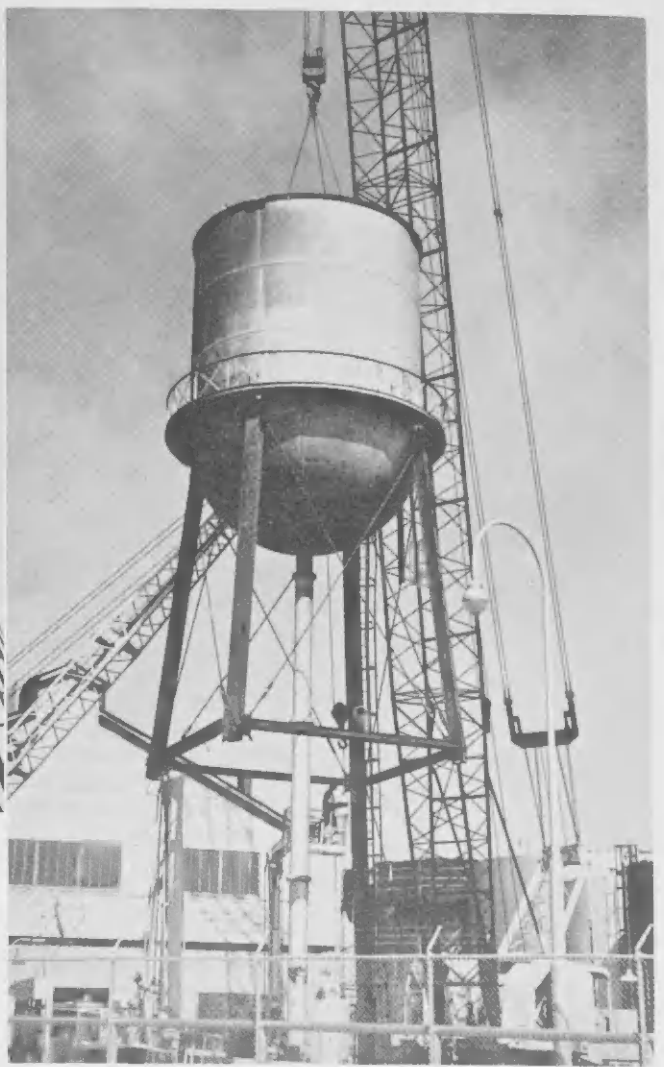
THREE WATER tanks were removed from the refinery skyline recently primarily through the efforts of the cutting torch. The tanks literally had their legs cut out from under them. In each instance, it would have been impractical, if not impossible, to pull them over. TRES TANKI di awa a worde kitá for di e silhueta di refinaria recientemente primeramente door di esfuernan di torcha cortador. Literalmente, e tankinan a haya nan pianan cortá for di bao nan. Den cada caso, lo tabata impractico, si no imposible, pa saka nan afor di ariba. Pesey nan a worde cortá.
